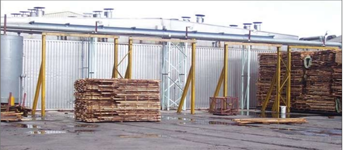
No spares or maintenance required on 206 Maxiflo units at Boskor, since installation in 2008
