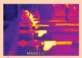
A thermal image of Maxiflo ejectors on hot plates at APL Cartons. Steam, presented in yellow, is held back in the equipment by the continuous discharge of condensate, presented in maroon.
